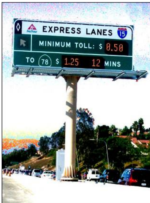
Figure 11. Dynamic Price Sign Installed in 2008 on I-15 in San Diego.
